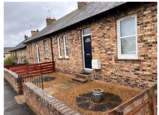
Right: renovated coal miner cottages in Cochrina Place, Roswell
